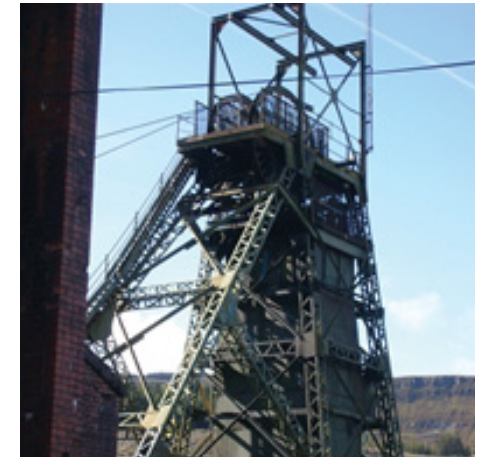
Above: Coal Mine Methane is extracted for health and safety reasons and then harnessed for energy creation.
