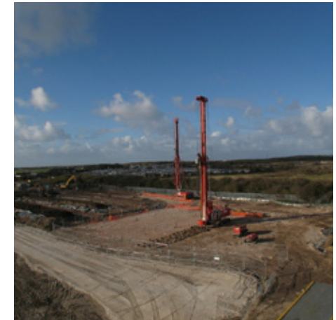
Above: Chemical oxidation by in-situ soil mixing on former chemical works.
